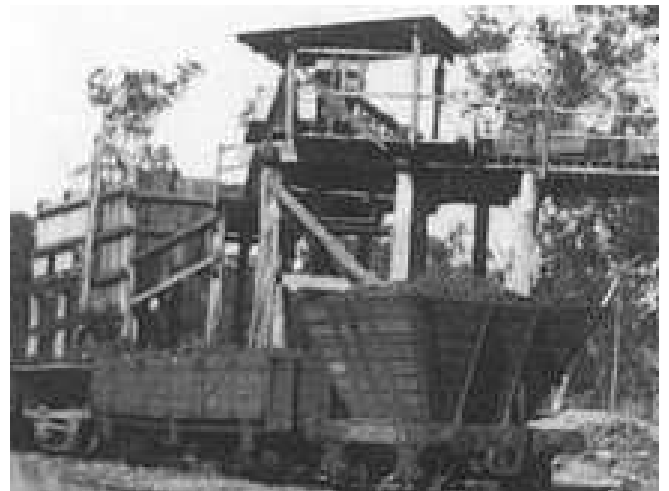
The raw Bunker sheathed ready for piers and walers to resemble this example in Qld.
